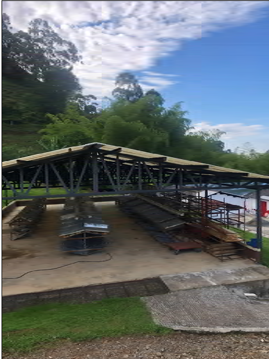
Figure 12-7 Core shed for core logging and sampling. (Source: Mauricio Castañeda, June 12, 2021)
